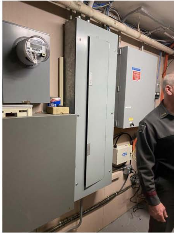
E-3 – Electric Meter and Main Distribution Panel
