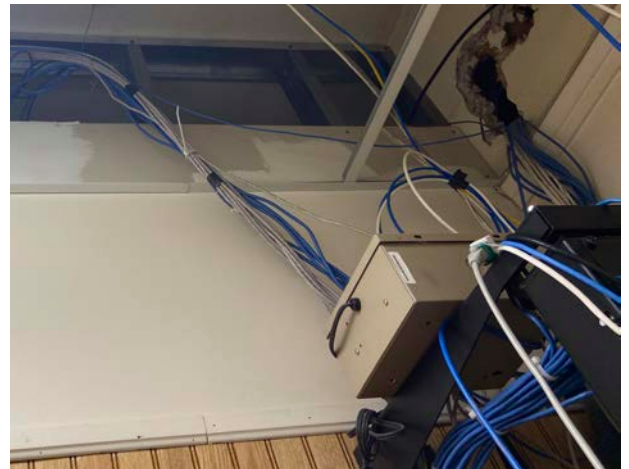
Non-compliant Wiring
