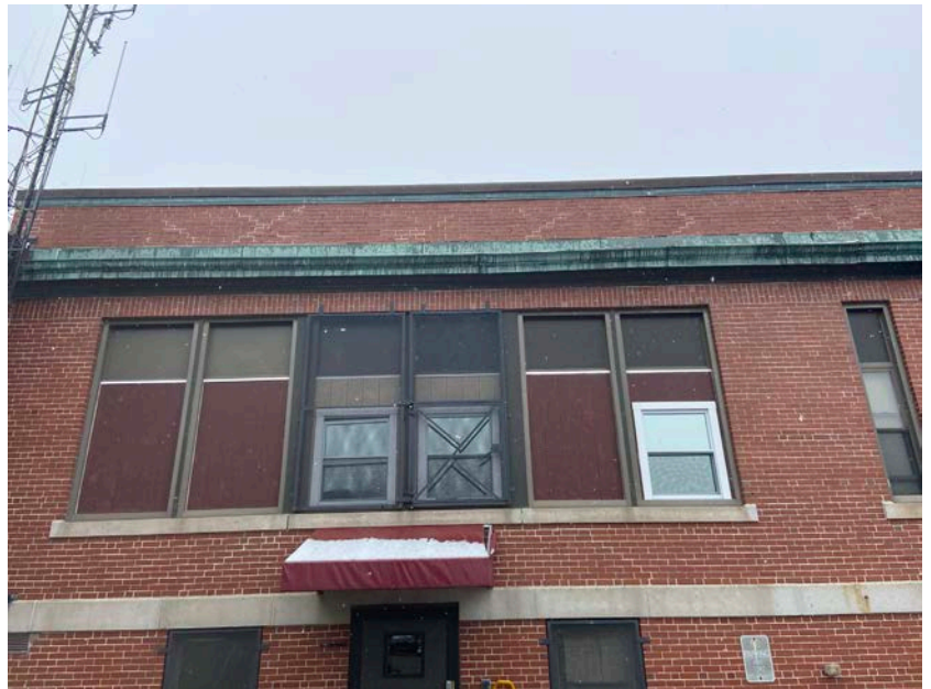
Vinyl Windows and Untethered Antenna
