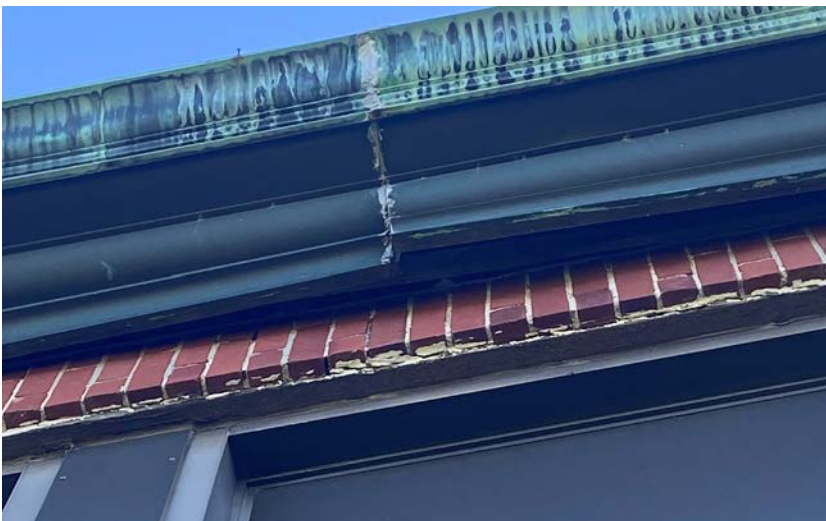
Copper Parapet Displaced by Masonry Failure
