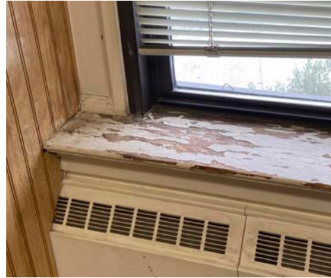
Water Damage at Exterior Wall
