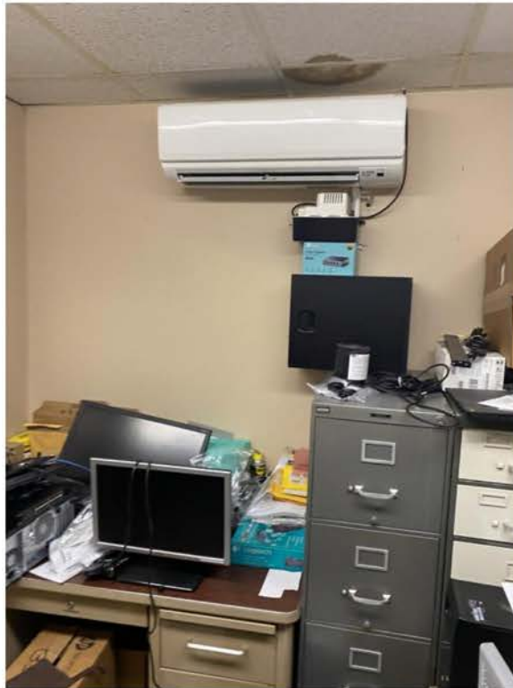
M-4 – Ductless Split Air Conditioner
