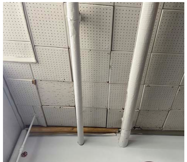
Wood Fiber Ceiling Tile Damage
