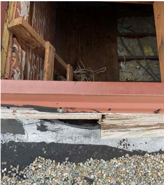
Gaps at Roof Hatch
