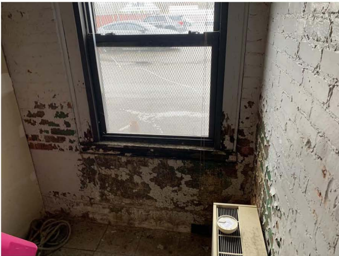
Interior Masonry Water Damage Photo #12
