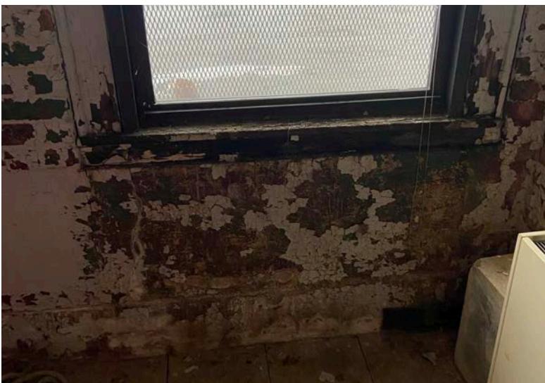
Mold and Moisture Damage
